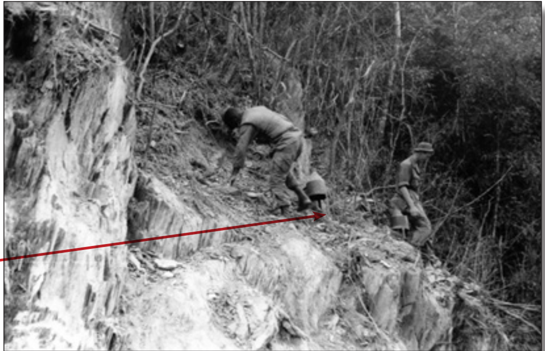
A/7 Engr 2nd Platoon Combat Engineers placing shape charges.
