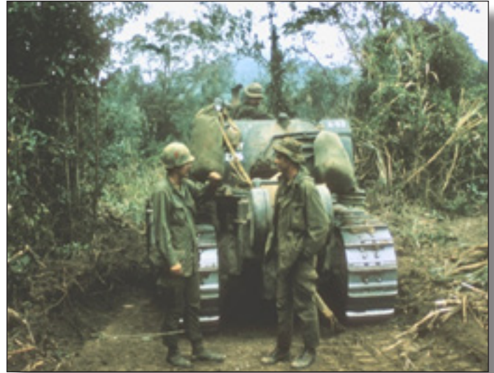
2LT Clinton Blick instructing a D7E team on clearing a path through the jungle (Red Devil Drive, west of Khe Sanh).
