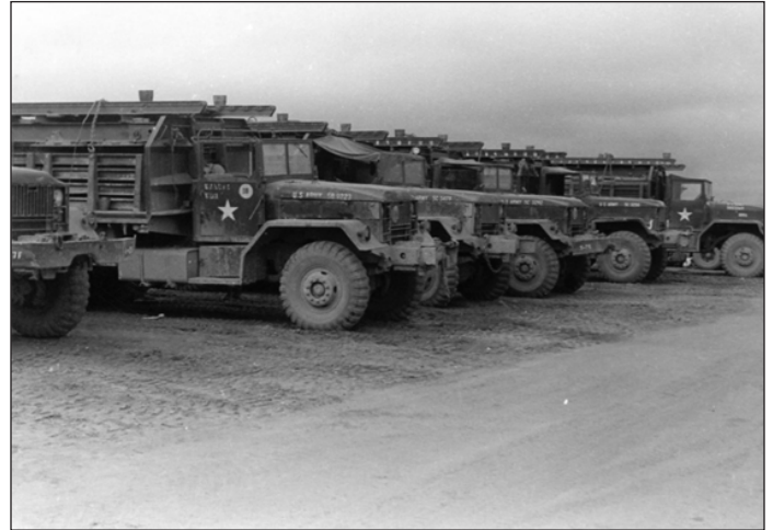
A/7 Engr bridge trucks were designed to be driven on terrain at and near water.
